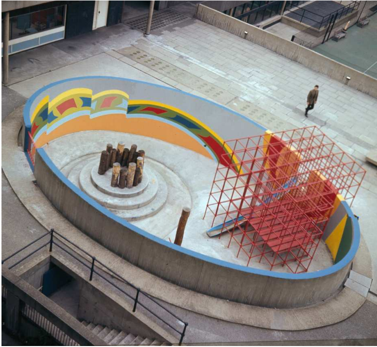
3/ Playground refurbishment undertaken in 1968, incl. significant alterations to the original wall (listed in 1997)
