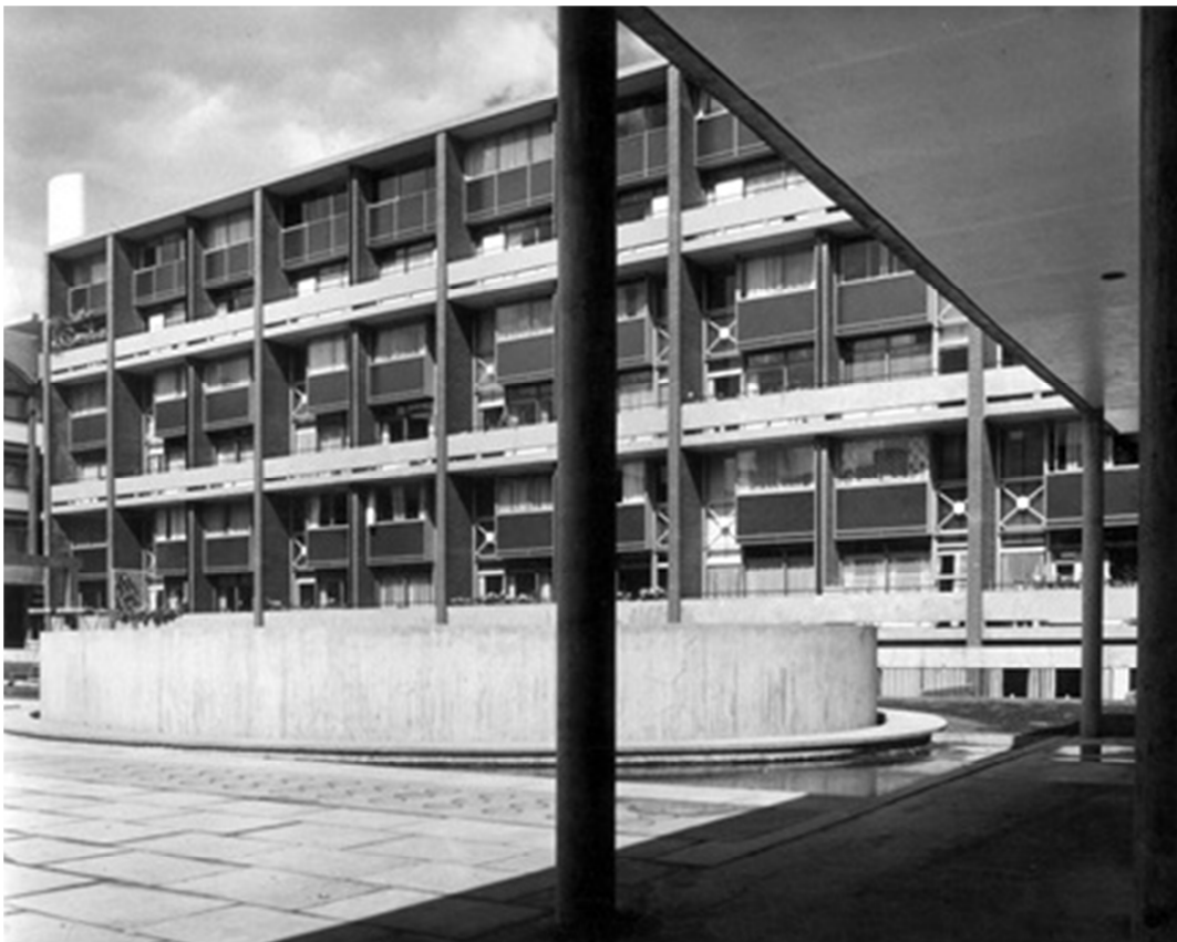
2/ Perimeter wall in 1962
